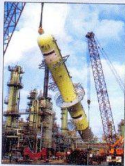
NARL reactor under installation
